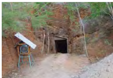
Entrance to No. 2 Tunnel.
